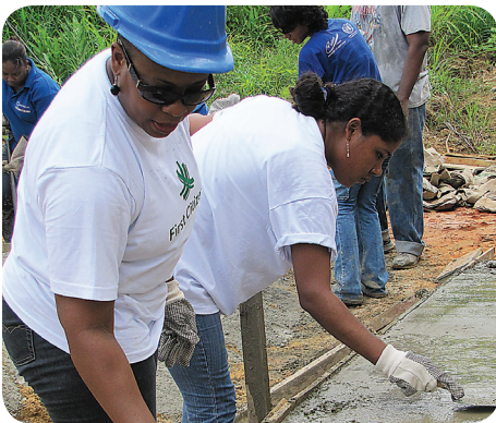
Staff undertaking plastering work
